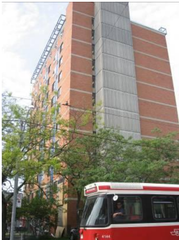
Green Phoenix Project
