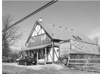
Photograph with tudor siding after alteration
