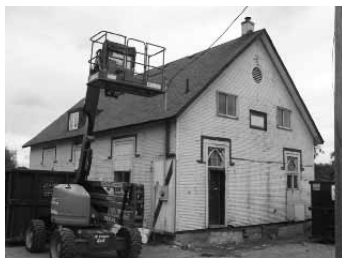
Photograph with white siding during siding removal
