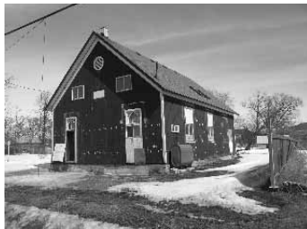
Photograph with red siding with original siding revealed
