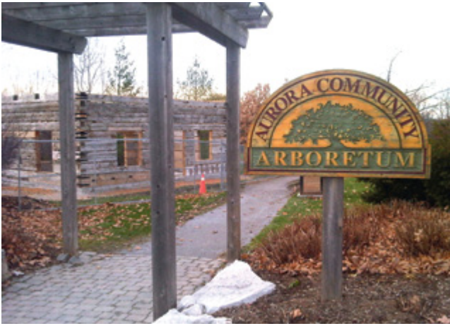
Petch log house being reassembled at the Aurora Arboretum on the banks of the East Branch of the Holland River
