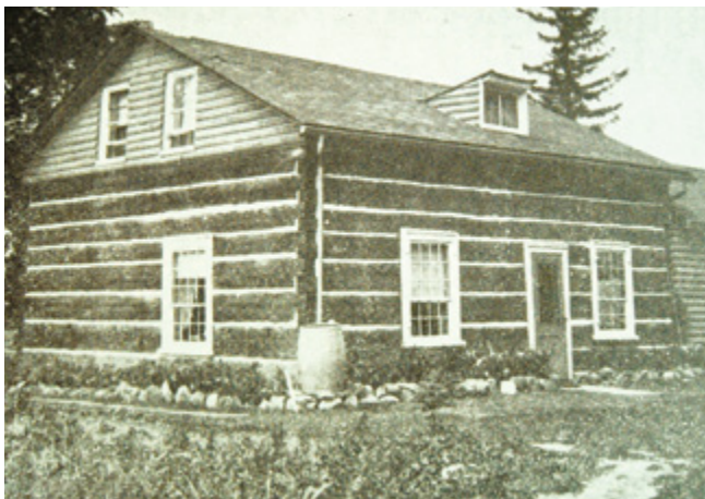
Petch House restored in the 1940s, with the assumption that the logs were originally exposed
