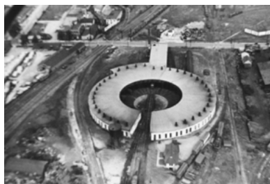
Former roundhouse/ New MBO Centre
