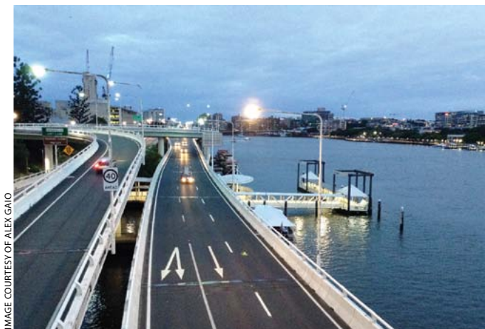
Riverside Expressway in Brisbane. Here, it's stacked on top of the Riverwalk
