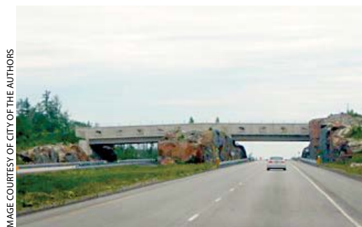
Ontario's new wildlife overpass on Hwy 69 south of Sudbury
