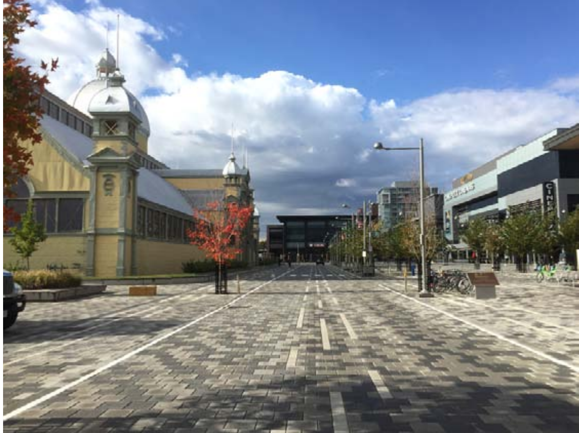
Contextual - old and new are combined harmoniously to create a new sense of place at Lansdowne Park in Ottawa
