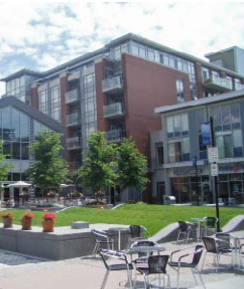
Diverse - fine grained mix of uses and housing types in St Lawrence Park, Port Credit
