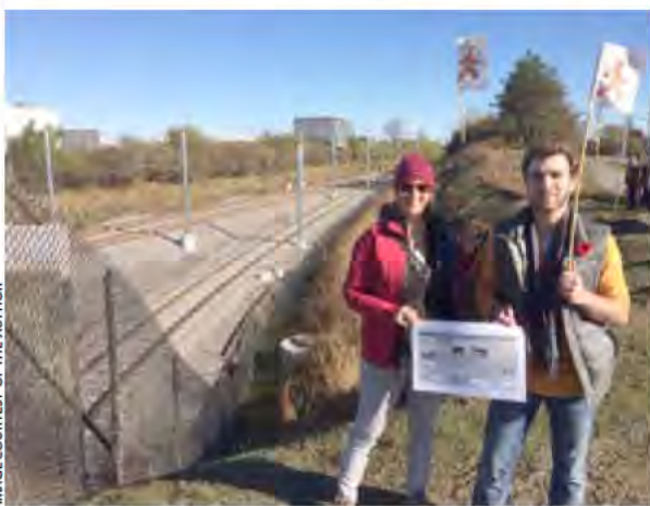
Thanks to Erin O'Connor and Eric Bays, here near the LRT line under construction, with their safety flags
