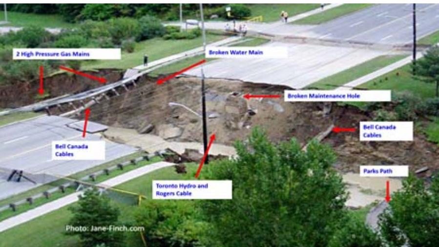
Toronto culvert washout that affected multiple infrastructure sectors
